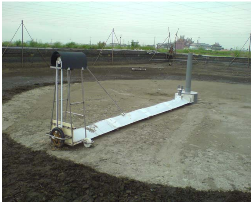
The sediment removing system
